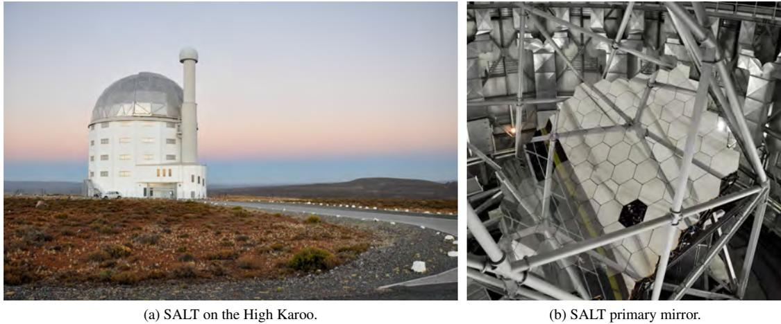
Fig. 1: The Southern African Large Telescope is located in the South African High Karoo desert near Sutherland. SALT is a 10 m-class, fixed zenith angle telescope with a spherical, multi-segmented primary mirror.
